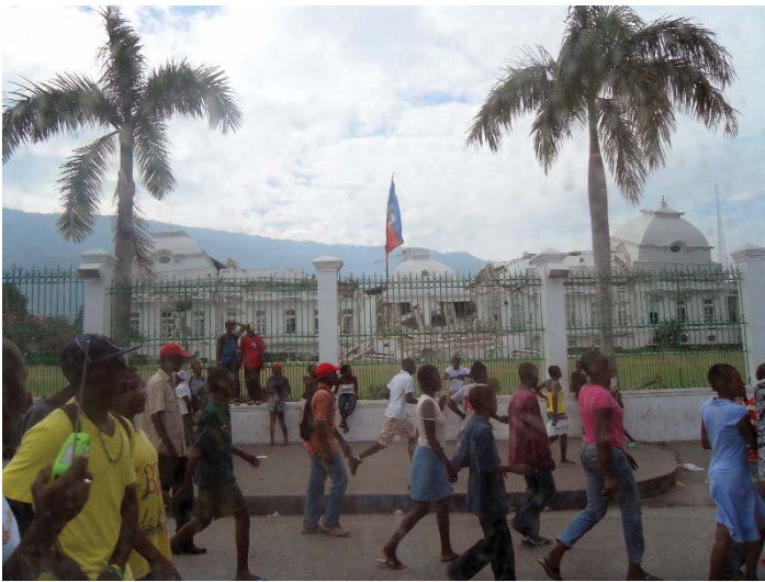
FIGURE 2. Post earthquake picture of the Presidential Palace courtesy of Dr. Reginald DesRoches
